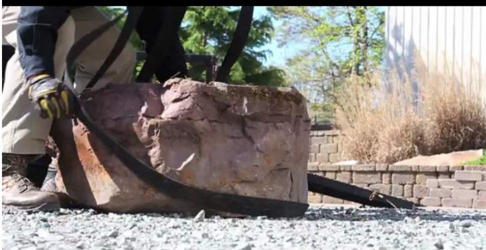
Engage the lift straps under the boulder
